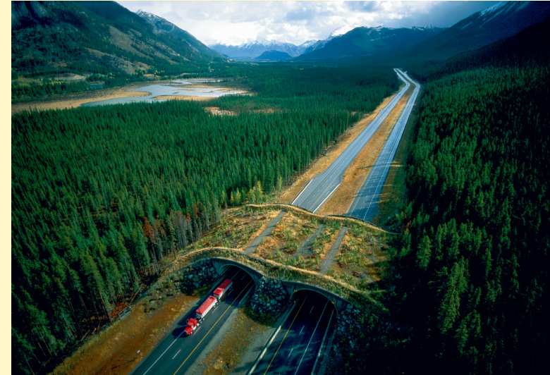
A wildlife crossing bridge built as part of the Banff Project.
